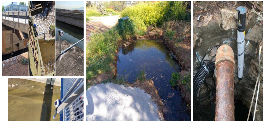
Installations of monitoring stations in: (i) Kifisos River, (ii) a selected monitoring well and (iii) construction of artificial wetland for pilot experiments at Athens Municipality Nursery.
